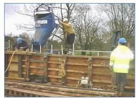
to hold it in while it is setting. After the concrete has set, the wooden structure is taken away and the concrete remains.
